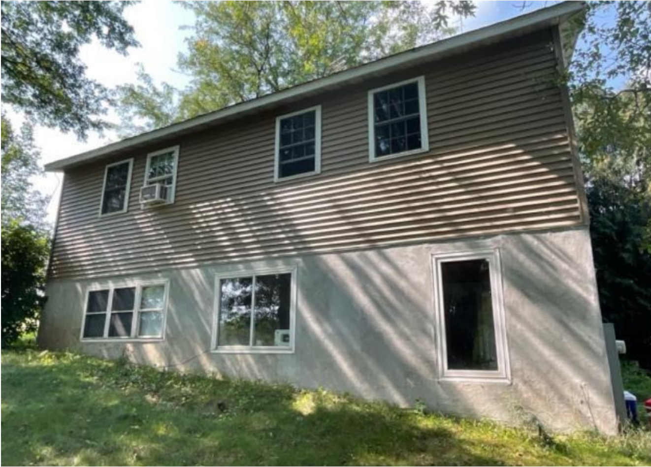
N9558 State Highway 69 and N9562 State Highway 69 on parcel 23024 0015.1000:
